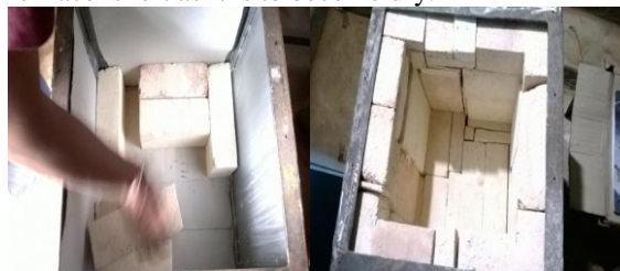
Fig 11 Stacking of refractory bricks inside the furnace frame
