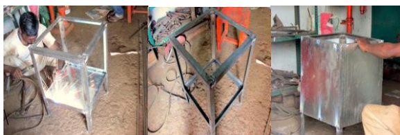
Fig 10 Construction of the frame of furnace
